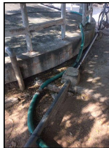
Connection to GP Bore well established
