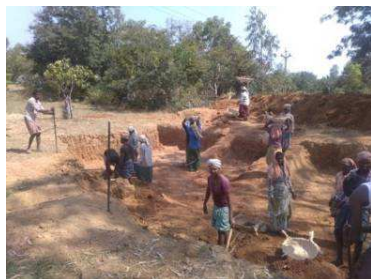
Digging Farm Pond
